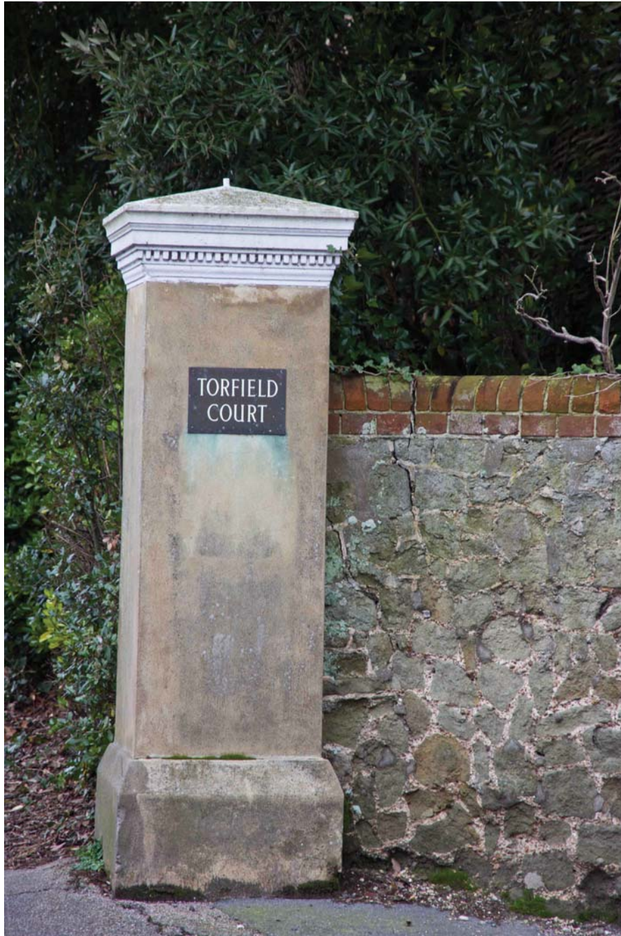
Picture 5 Torfield Court pier, St Anne's Road.
