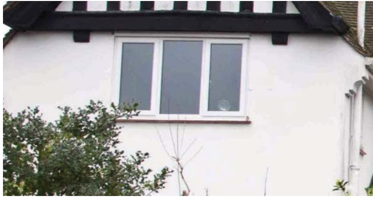
Picture 19 UPVC replacement windows.
