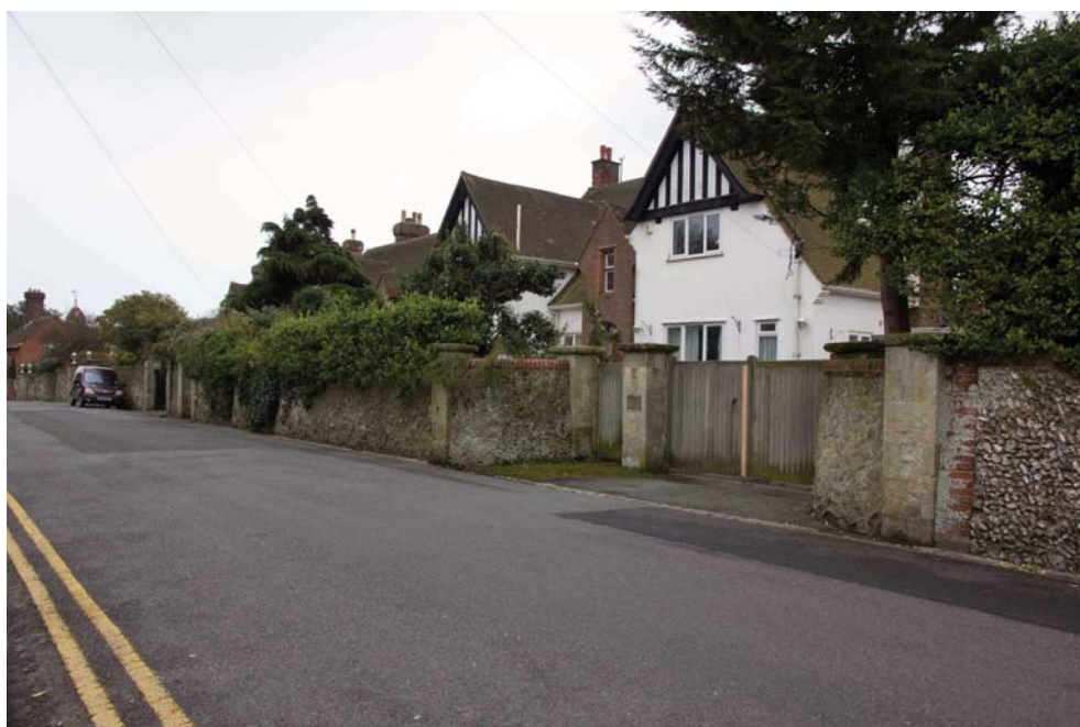
Picture 17 Dorset House, St Anne's Road, greensand piers and boundary walls.
