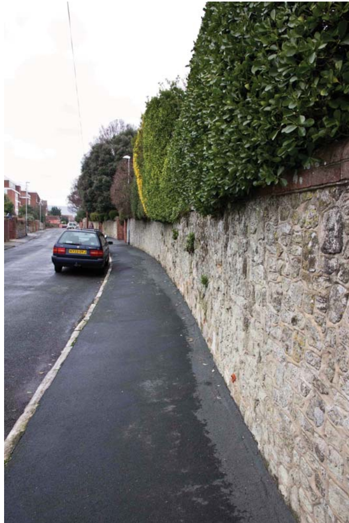
Picture 2 Selwyn Road, boundary walls.
